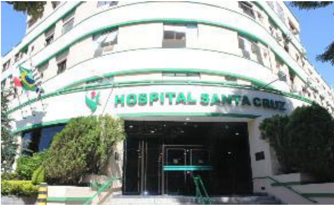
Fachada do Hospital Santa Cruz – São Paulo (SP)
